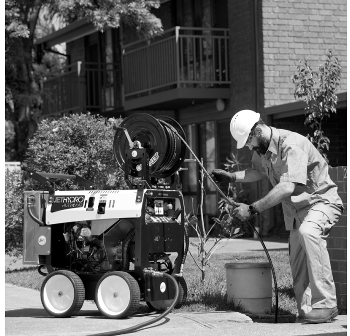
Figure.7 - Extending the Drain Opening to the Operation Point
