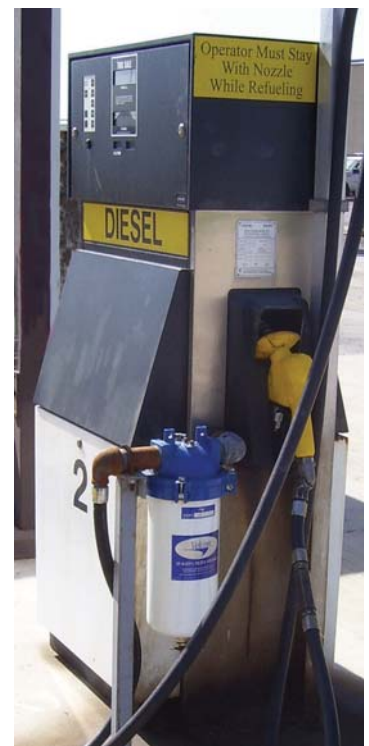
VF-61 connected to a diesel fuel dispenser
